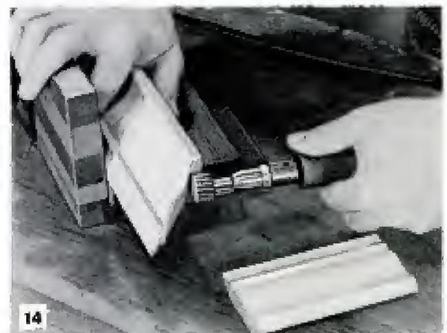
Some workmen prefer to undercut the cope with a rotary file, or burr, driven by means of a hand grinder
